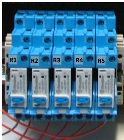
Figure 68 Relay Outputs
